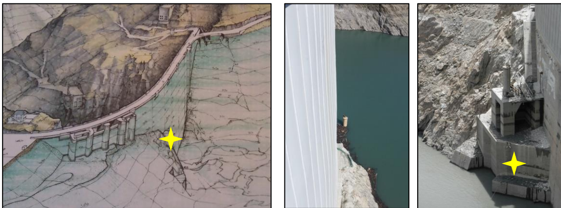
Figure 10 Examples of installation at a hydroelectric dam
