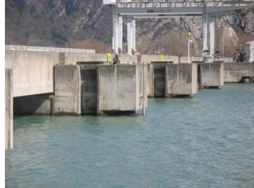
Figure 1 Bathyswath-2 PSM At a Run-of-River Hydroelectric Site
